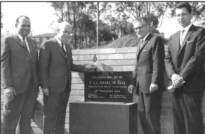
President of the Baptist Union N.A. Wales, F.J. Church with Architect H.R. Hodges Snr and builder F.C. Zadro laying the foundation stone at Waldock
