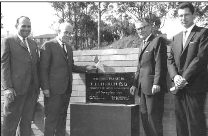
President of the Baptist Union N.A. Wales, F.J. Church with Architect H.R. Hodges Snr and builder F.C. Zadro laying the foundation stone at Waldock
